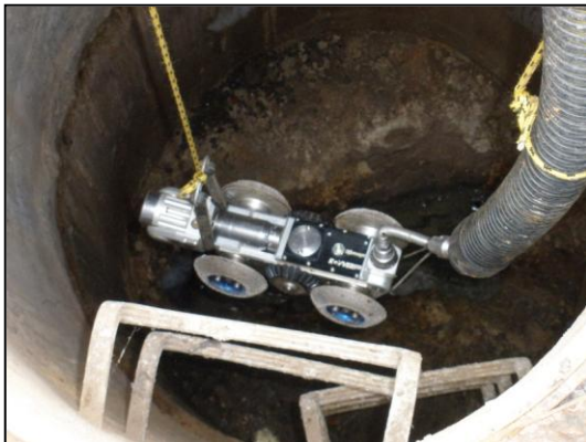
Tractor mounted camera being lowered into a manhole to access the main line.
